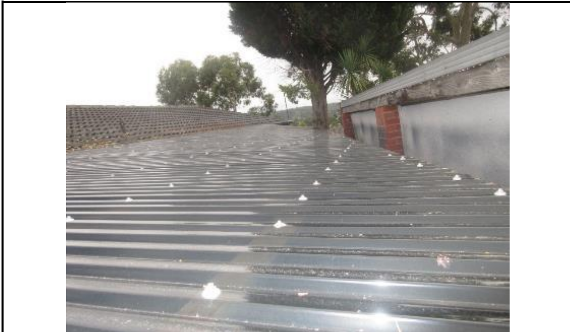
Photograph C1. View of verandah roofing.
