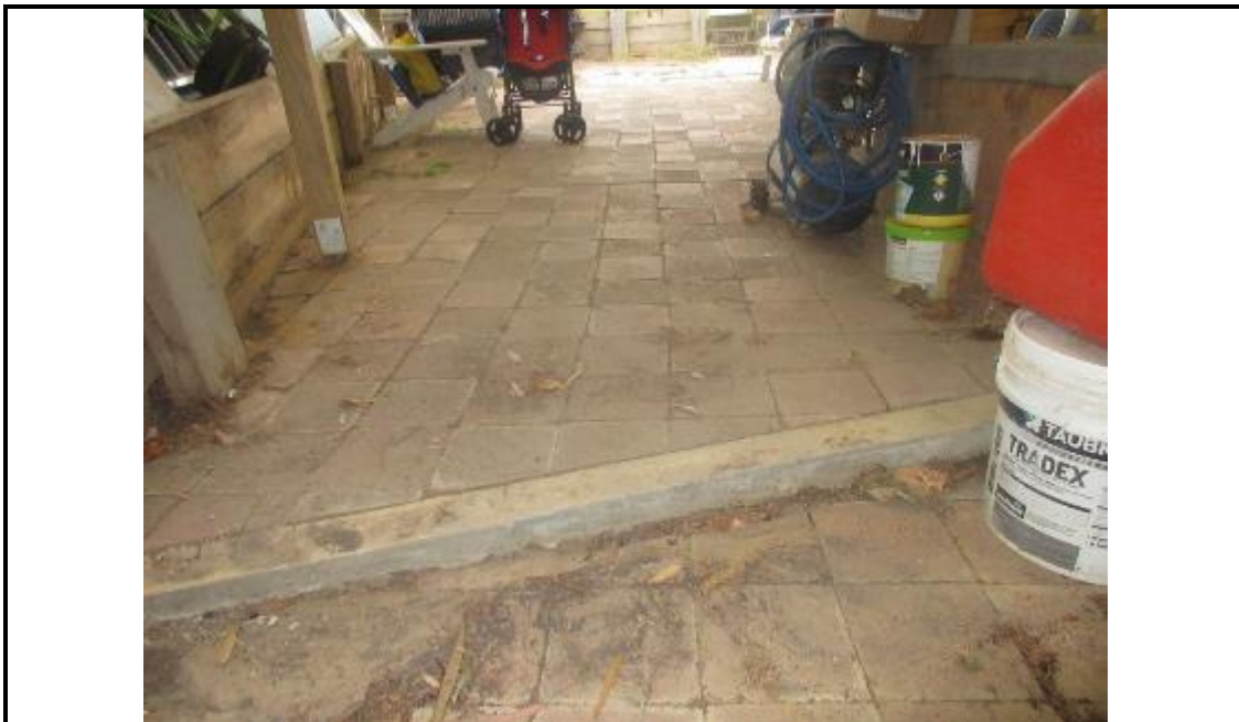
Photograph B2. View of unit pavers.
