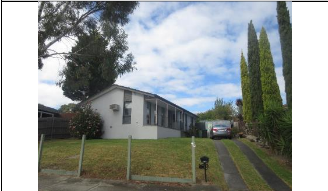
Photograph 1. View of front of residence.
