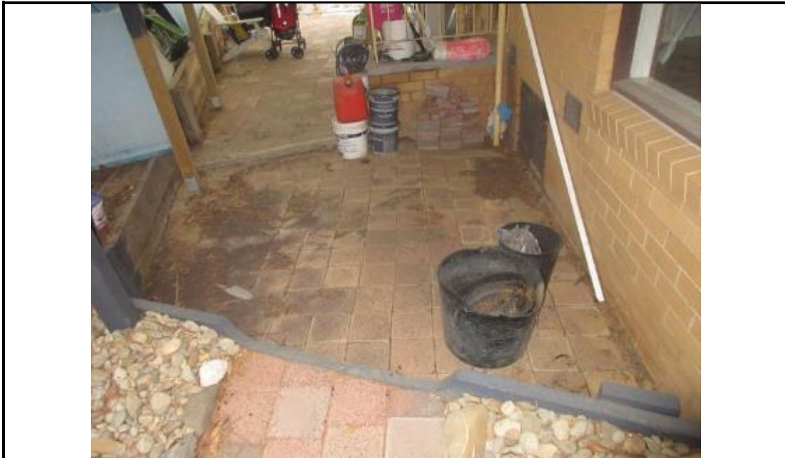
Photograph B1. View of unit pavers.
