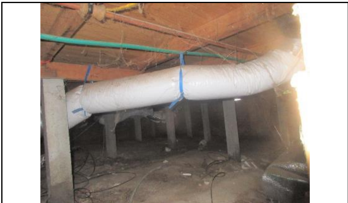
Photograph 16. View of sub-floor space.
