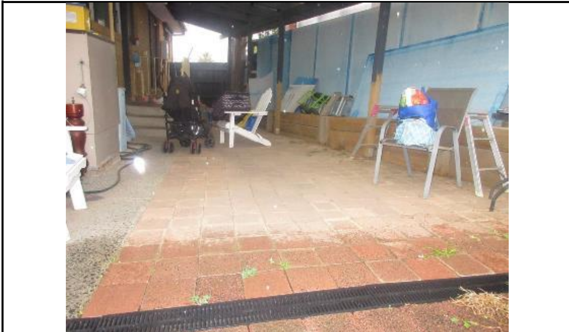
Photograph B3. View of unit pavers.
