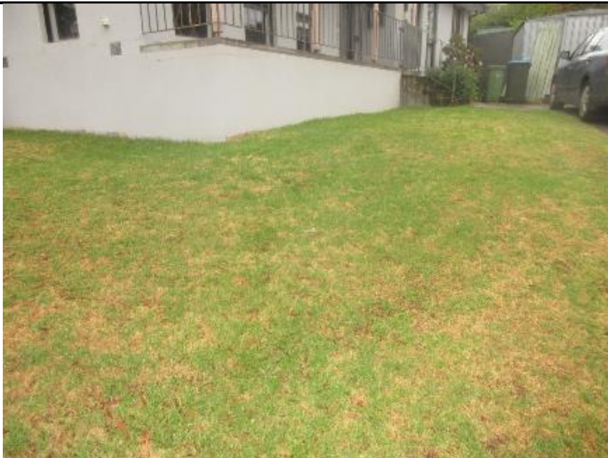
Photograph 17. Broken and leaking stormwater drain located downhill of north-west corner of residence.
