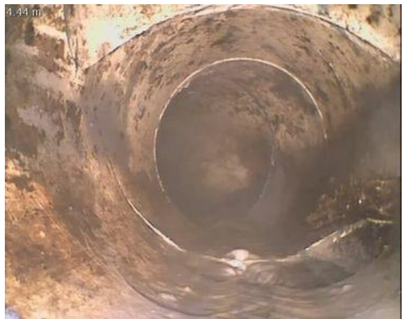
CCTV OF DRAIN
