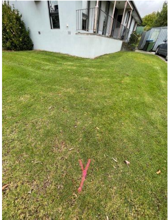
DIG AND REPAIR STORMWATER AT THIS POINT
